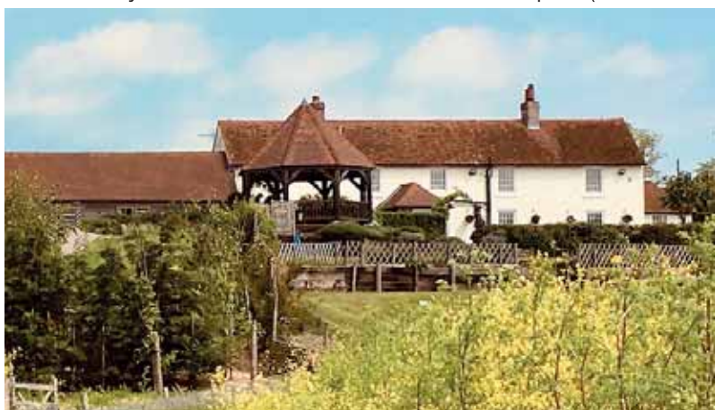
The Ferryman’s Inn at Harty, Isle of Sheppey (a grade II listed building)
