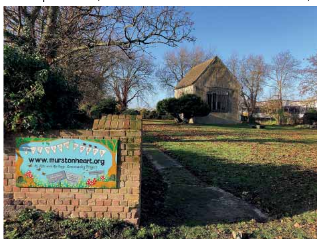
Murston Old Church – a Scheduled Monument with the project to repair and re-use the church supported by the Council.
